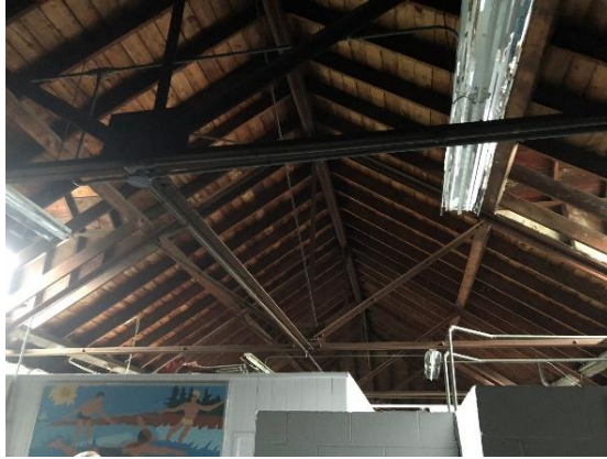
Steel truss/wood deck structure
