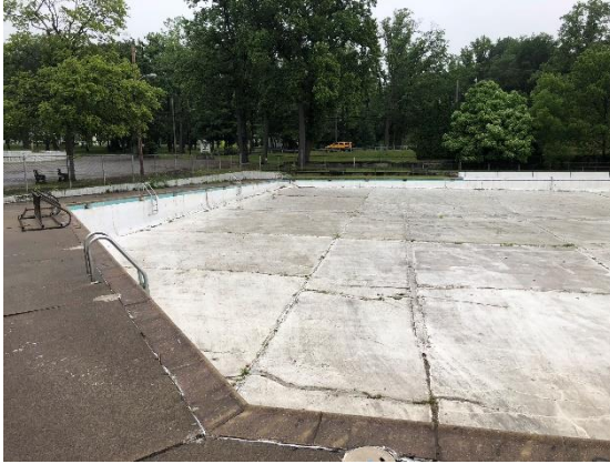
Main pool floor structure
