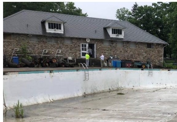
Bathhouse structure - exterior looking north-east
