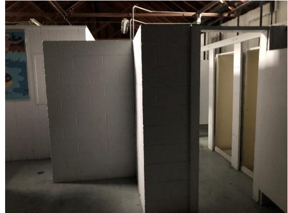
Interior circulation – Shower
