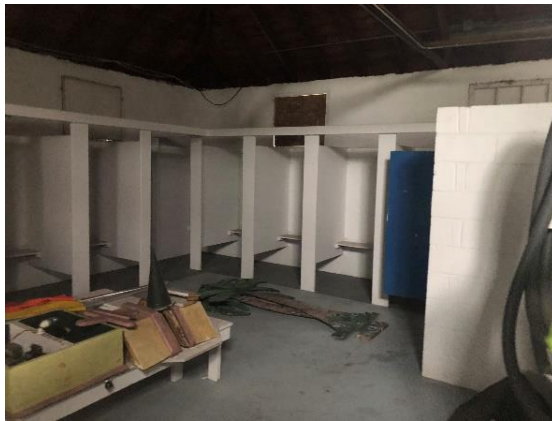
Interior dressing area - Storage
