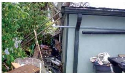
Accumulation of rubbish or garbage
